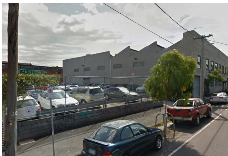
View looking north-east from the Little Nicholson Street and Mollison Street intersection.
