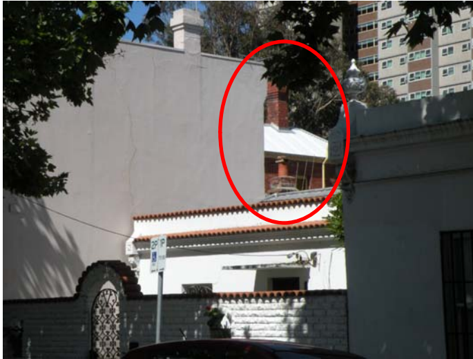
Above : Extent of existing rear wing that is currently visible from George Street shown circled
