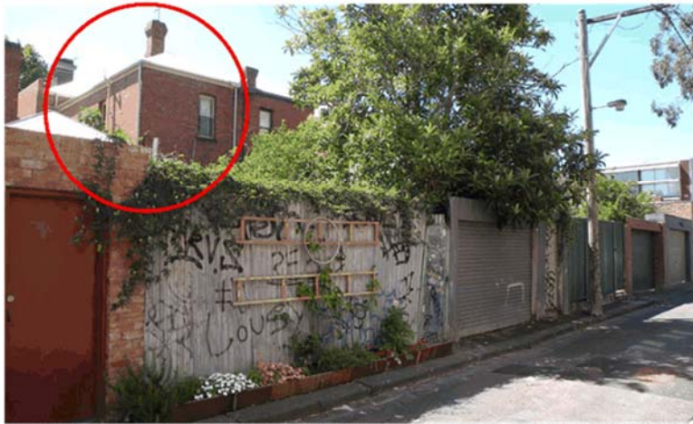
Above: Extent of existing rear wing that is currently visible from Little George Street shown circled
