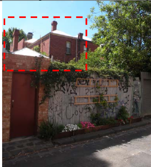
Above: Rear of subject site.
