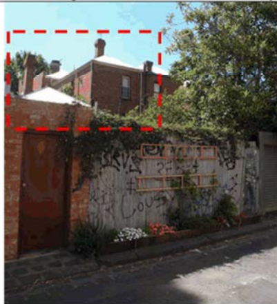
Above: Rear of subject site.
