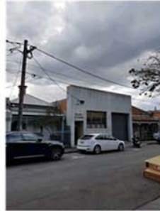
Existing Photo 01 Howard Streetscape
