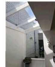
View Towards No.17 Light Court Facing South
