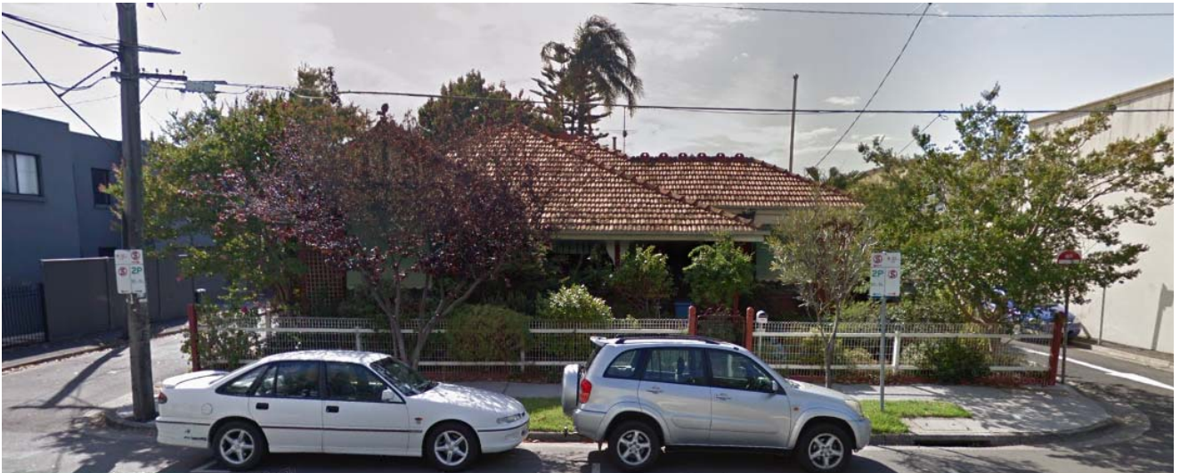
Coppin Street façade
