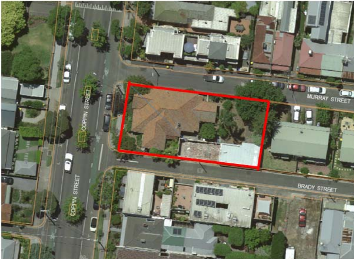
Figure 2 – Aerial photograph with subject site outlined
