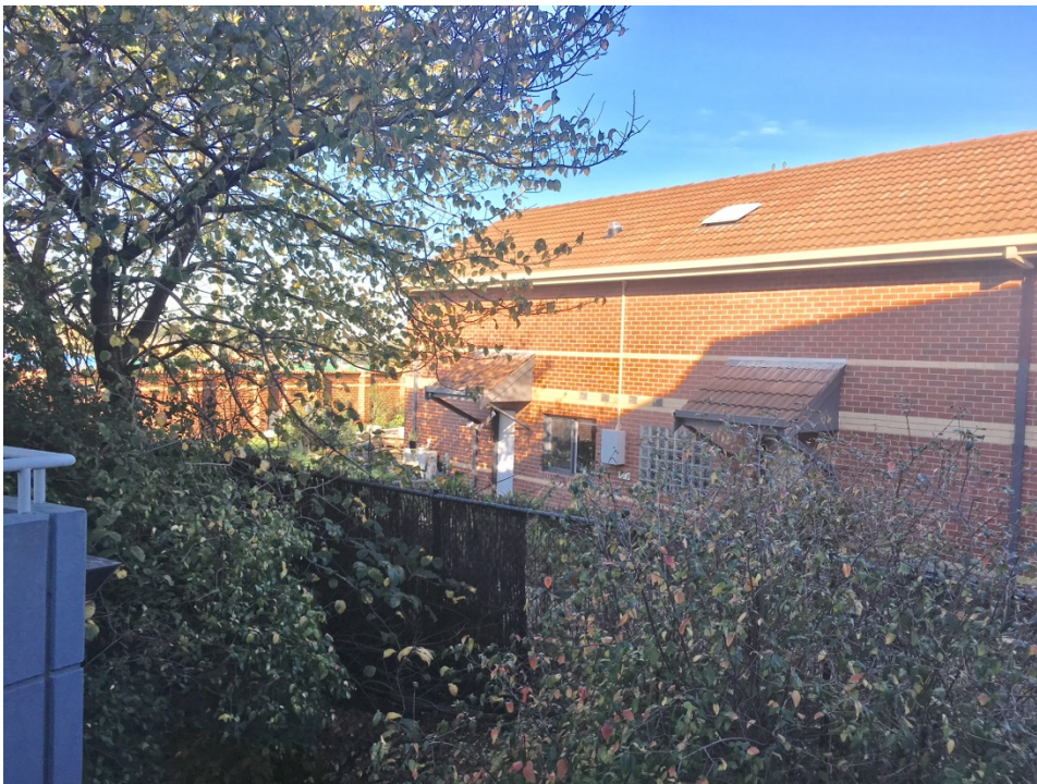
Northern elevation of the townhouse to the south at 35 Coate Avenue
