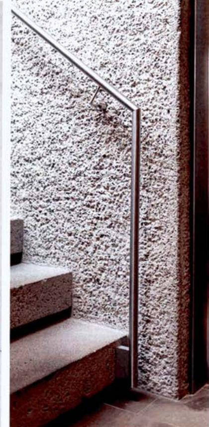
BUSH HAMMERED CONCRETE WALL - Battersby & Howat Architects
