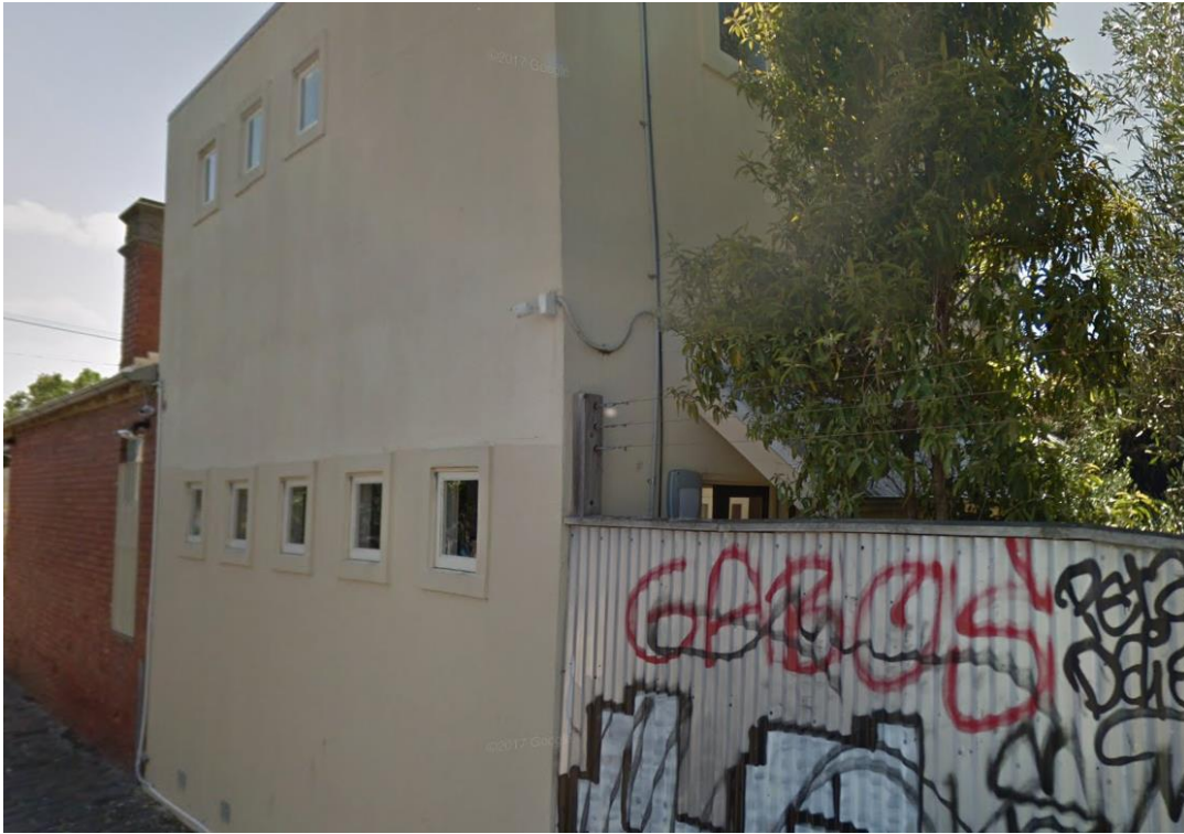
Western wall and HRW of No. 100 Leicester Street
