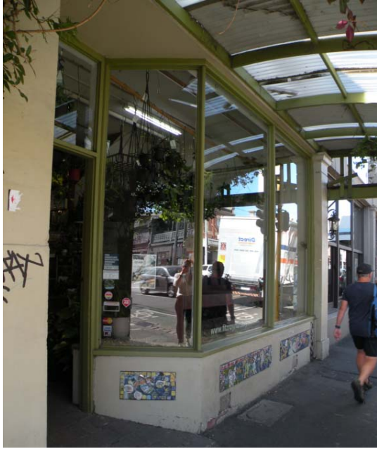
Left: Existing shopfront
