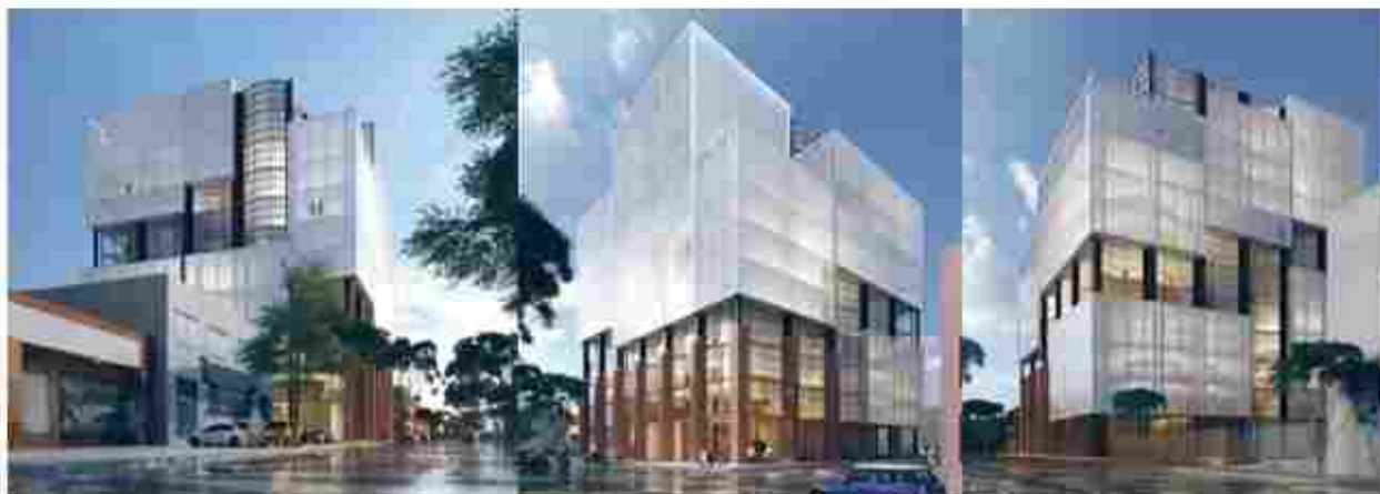
Looking from the north, southward along Nicholson Street
