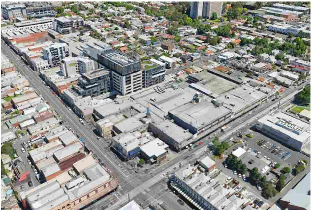
(Looking north – west along Bridge Road)
