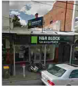
#2. 217 SWAN STREET ONE STOREY BRICK OFFICE
