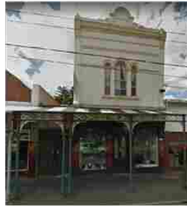
#3. 219A SWAN STREET TWO STOREY RENDERED BRICK SHOP
