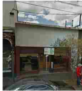
#4. SUBJECT SITE - 221 SWAN STREET ONE STOREY BRICK SHOP
