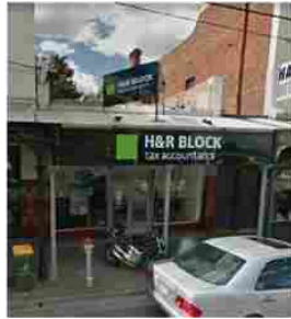
#2. 217 SWAN STREET ONE STOREY BRICK OFFICE
