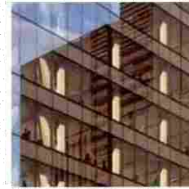
Structurally glazed curtain wall with integrated shadowbox, spandrel panel FT01, FT02, FT03
