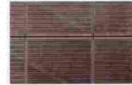
Tower - bronze metal mesh screening FT09
