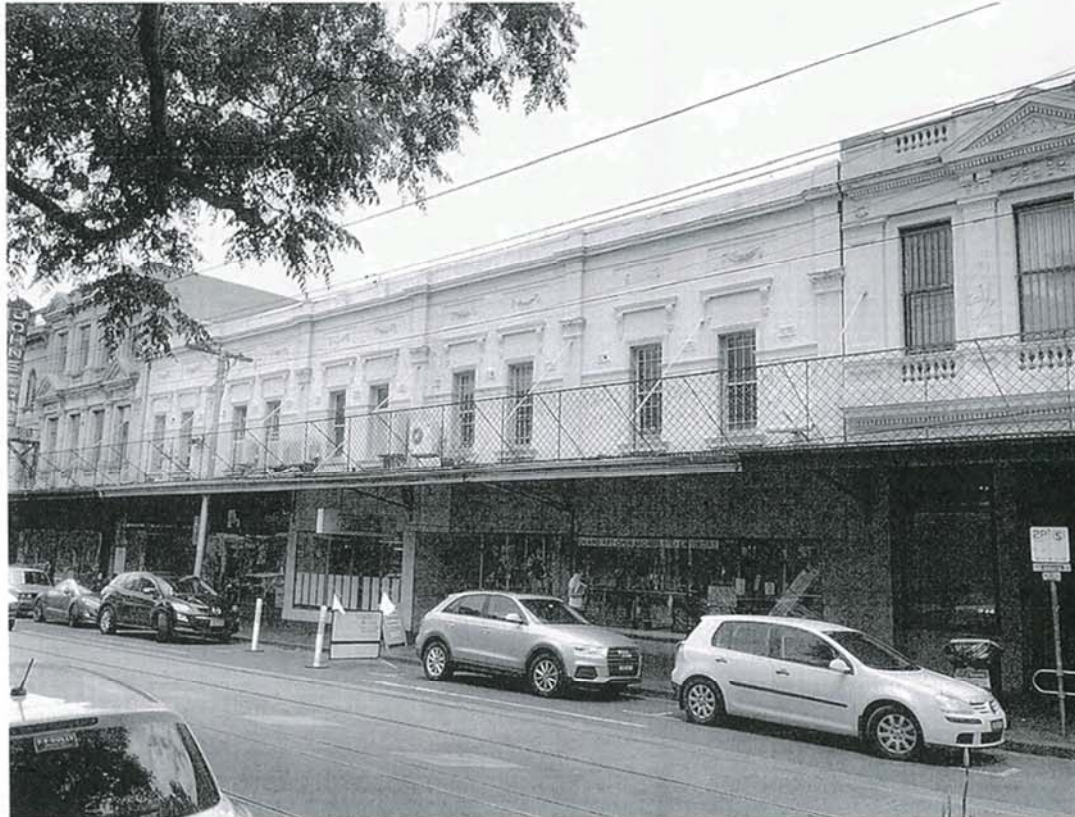
Proposed minor facade and access upgrade to existing heritage building 188-196 Gertrude Street Fitzroy Victoria 3065
