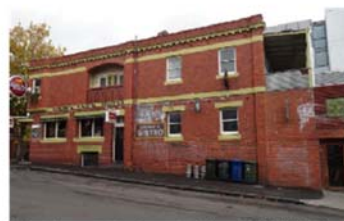
View of property to the west of the site in Webb Street
