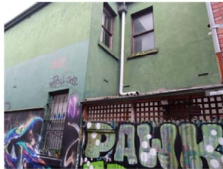
View of existing windows from the laneway
