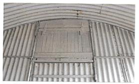
Figure 7 Detail of opening & door, east elevation. Note original timber infill above
