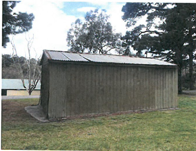
Figure 14 Detail of existing Shed 3 showing concrete slab
