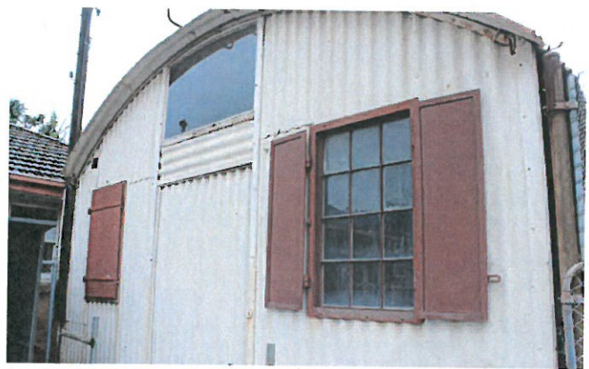
Figure 3 Detail of West Elevation.
