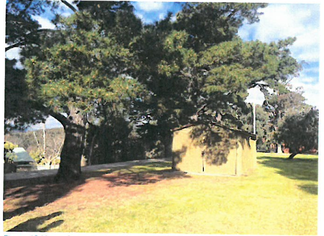
Figure 12 View of existing Shed 3 and the existing context
