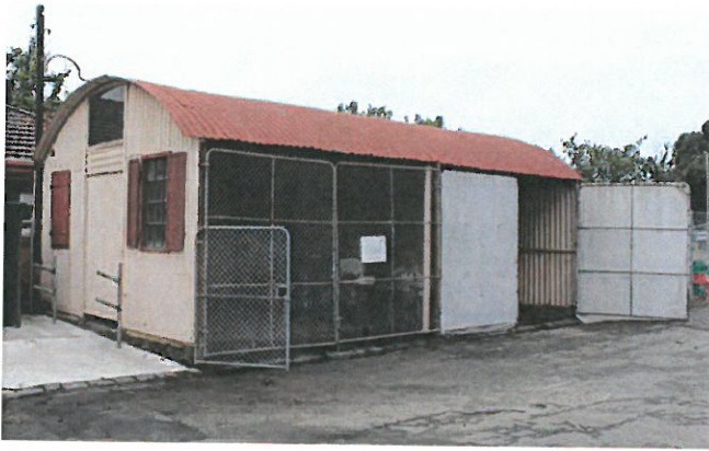
Figure 2 South & West elevations. Note replacement gates on south elevation.
