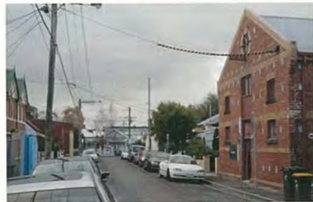
'The Stables' 19 Duke Street Shows composite form addressing residential fine grain street
