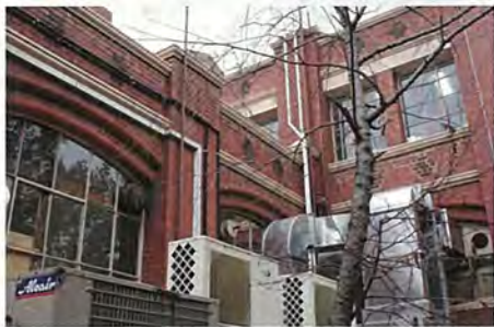
Existing Heritage Courtyard of Wertheim Building
