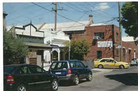
Metzke Bros, 89 Type Street Composite industrial forms at block corner, contrasting with fine grain residential. Variation in composite form.
