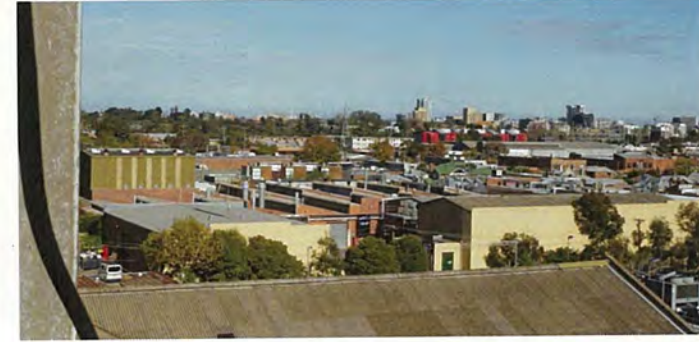
06/ VIEW LOOKING SOUTH FROM TOWER RL. 40.7
