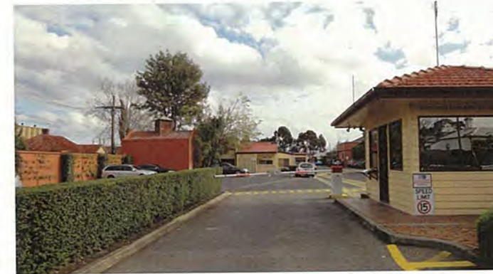
14/ GATEHOUSE MAIN ENTRY FROM BENDIGO ST
