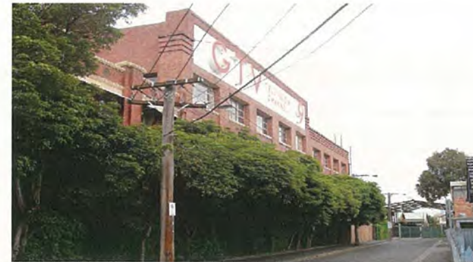
02/ LOOKING WEST ALONG JAGO ST
