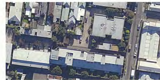
SOUTHERN END OF TYPE ST AT HOFERT LANE
