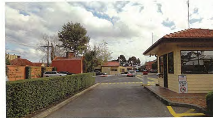
14/ GATEHOUSE MAIN ENTRY FROM BENDIGO ST
