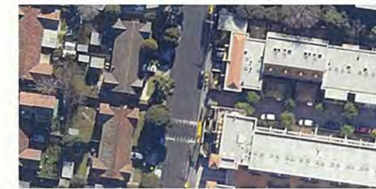
WESTBANK TERRACE NORTH OF CAMPBELL ST JUNCTION
