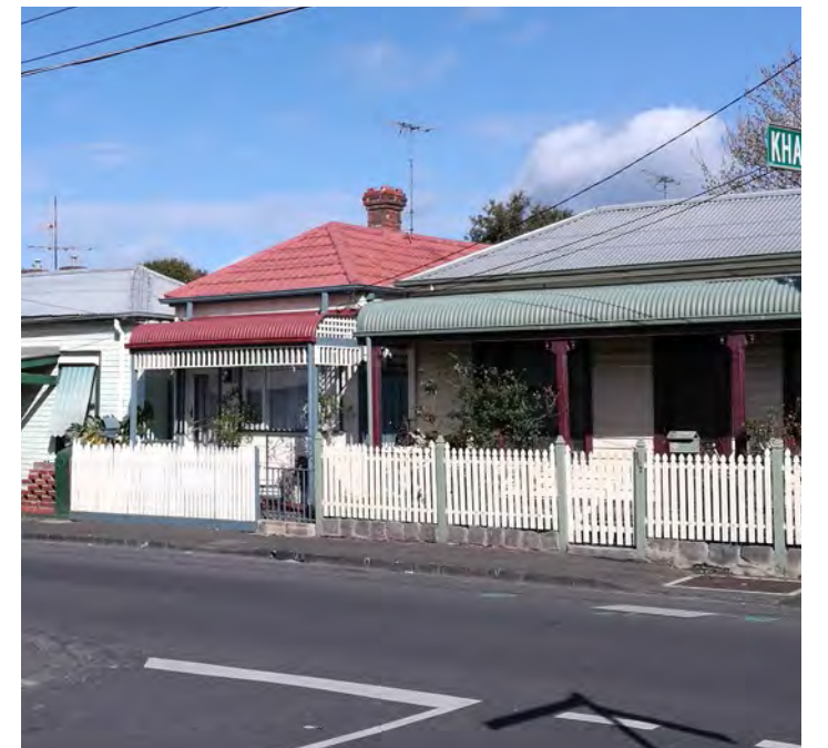
Contextual street frontage character
