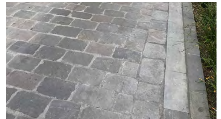
Cut heritage bluestone cobbles to carriageway between Blocks B and E
