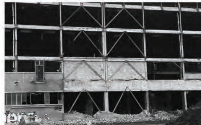
THE PAPERMILL DIAGONAL STRUCTURE
