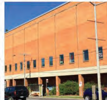
EXISTING HEIDELBERG ROAD FACADE
