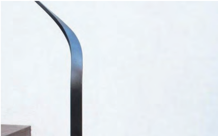
Steel Handrail Return
