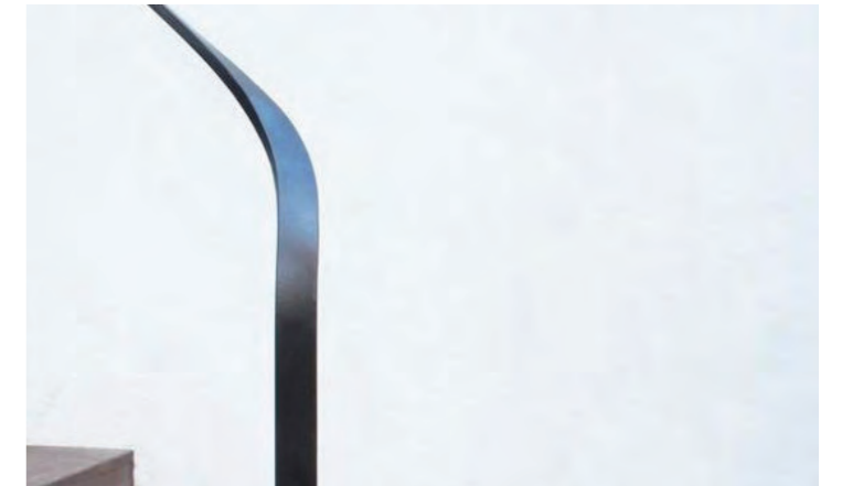
Steel Handrail Return
