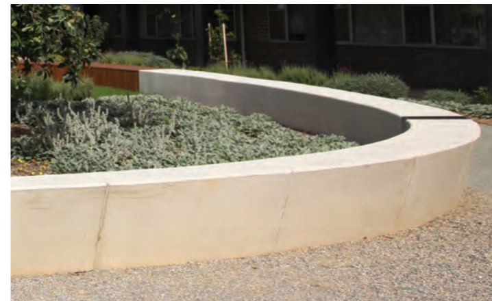
Concrete Seat Wall
