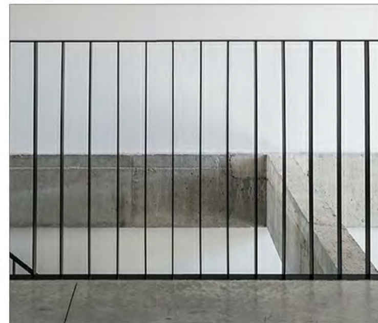
FM-02 STEEL FLATS BALUSTRADE POWDERCOATED FINISH
