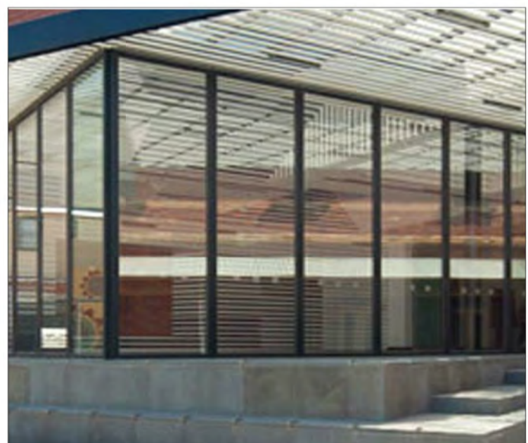
GL-03 SHOPFRONT CLEAR GLAZING POWDERCOATED FINISH
