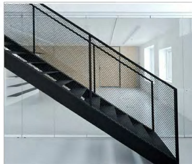
HR-05 STEEL STAIR + BALUSTRADE POWDERCOATED FINISH
