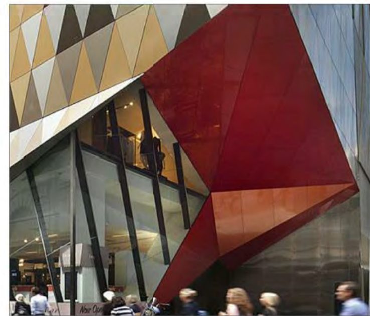
CD-03 ALUMINIUM COMPOSITE PANEL POWDERCOATED FINISH
