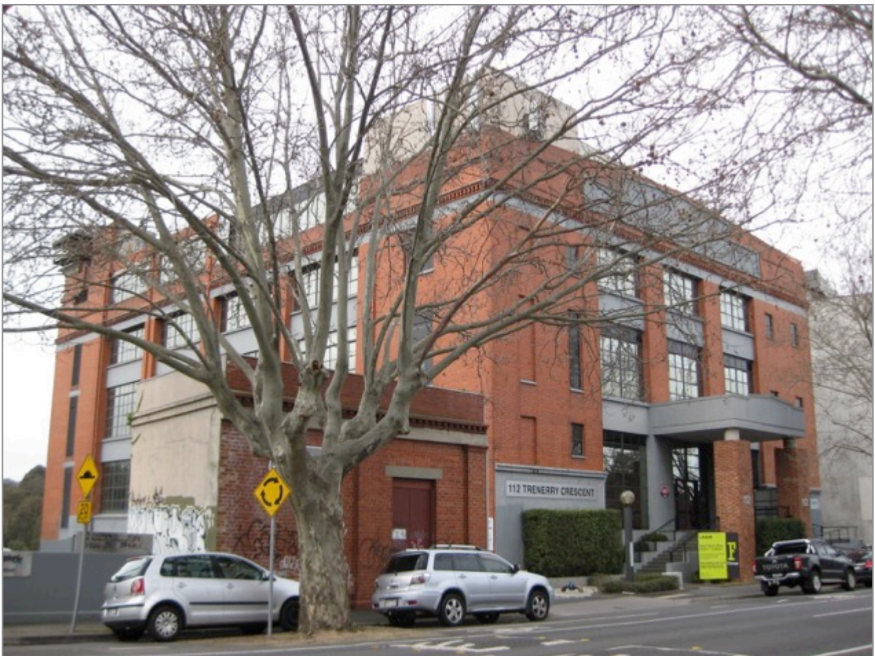
Figure 1. 112-124 Trenerry Crescent, Abbotsford: the main four-storey building and the remaining section of a contemporary building to the north (foreground) (2016).
