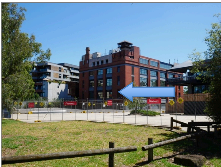
Figure 15. 112-124 Trenerry Crescent – from Dights Falls Reserve (arrow indicates maximum height of new built form to the east) – Figure 22 from Mr Gard’ner’s evidence.
