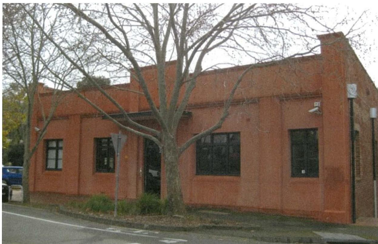
Figure 1. 20-60 Trenerry Crescent, Abbotsford: the facade of the 1911 building.
