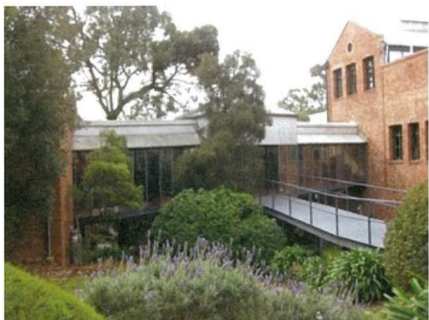
Figure 2. The north-west elevation of the 1911 building (right) with its gabled third-storey, the 1984 glazed walkway and the modified 1920s brick office building (left).
