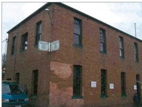
Figure 11. Rear of 16 Arnold Street, Princes Hill (©Google)
