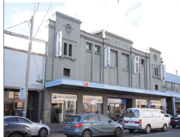
The former Austral Theatre, 200-202 Johnston Street, Collingwood (Source: Context Pty Ltd, 2015)
