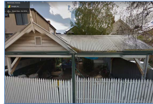
Rear of 283 Punt Road
