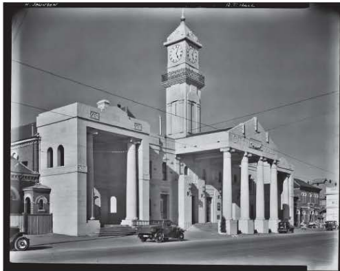
Figure 10. The City Hall after the remodeling, photo taken late 1930s (SLV Image no. H2009.20/12).
