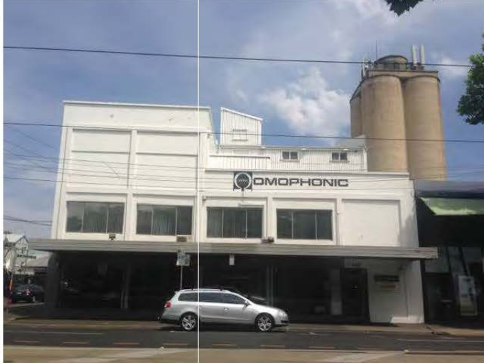
Bridge Road elevation
