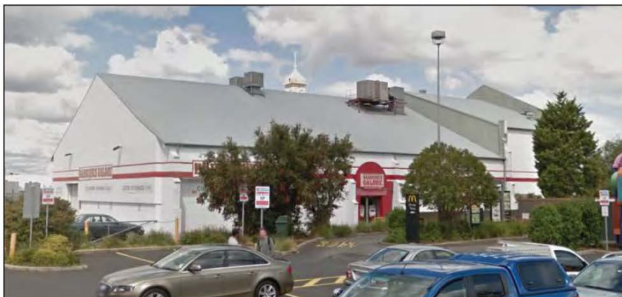
Figure 18. 311 Bridge Road (rear), Richmond (May 2018)
