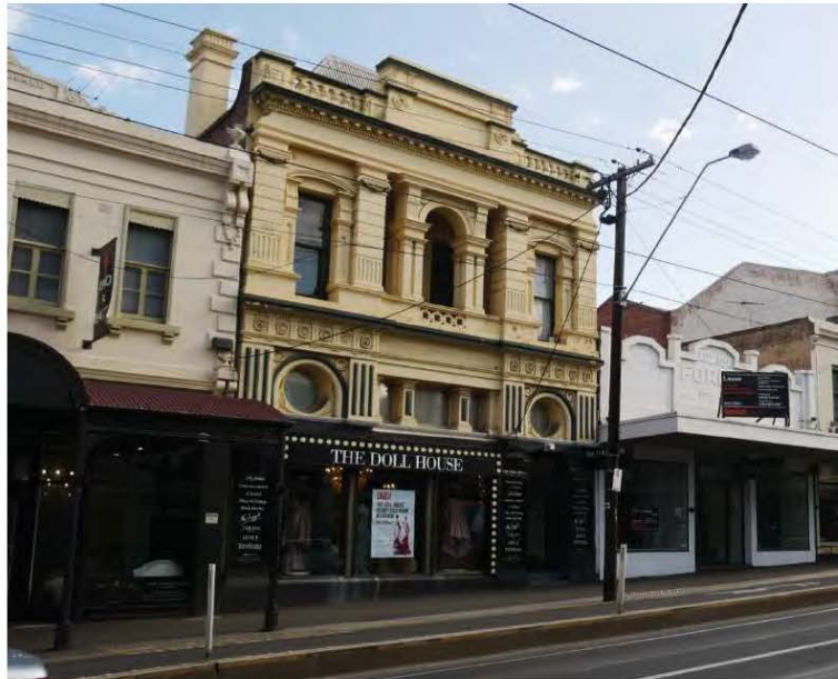
Figure 1. 184 Bridge Road, Richmond (GJM Heritage, September 2017)
