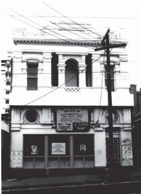
Figure 5. The building in 1985; painted, with an altered ground floor facade (O'Connor et al, 1985: building identification form).
