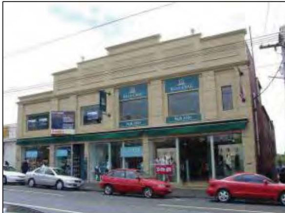
Figure 7. Former Nation Picture Theatre before demolition (VHD image)
