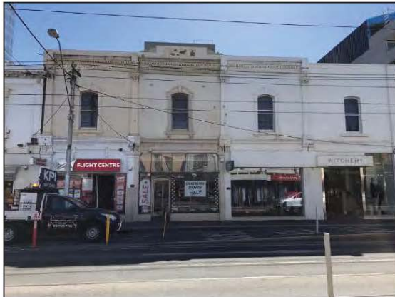
Figure 8. (Left to right) 109, 111, 113 & 115 Bridge Road (GJM Heritage, February 2018).
