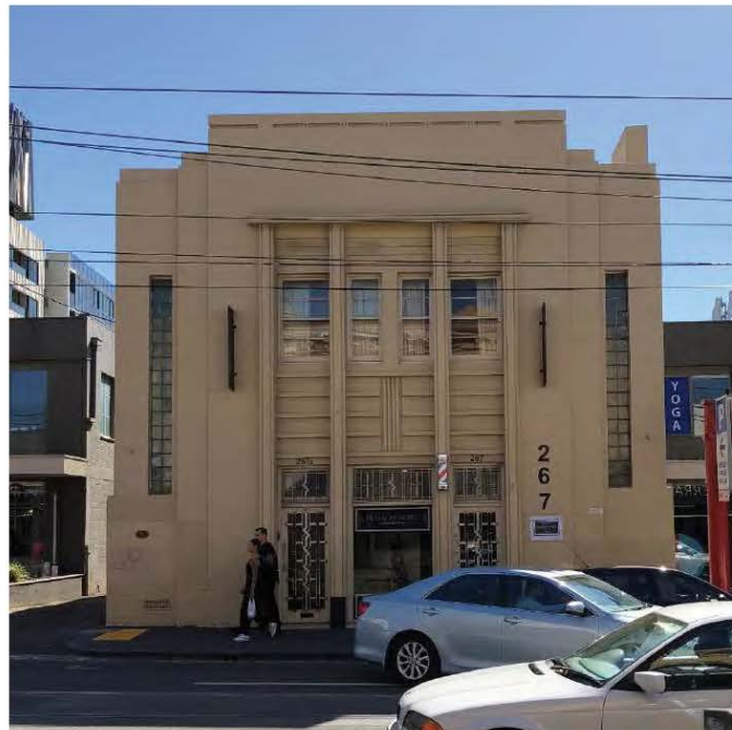
Figure 1. 267 Bridge Road, Richmond (GJM Heritage, September 2017)
