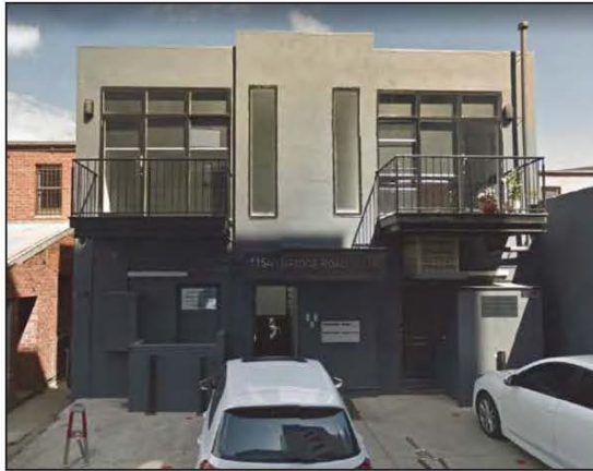
Figure 9. (Left to right) 115A & 113A Bridge Road, facing Corns Place (©Google).
