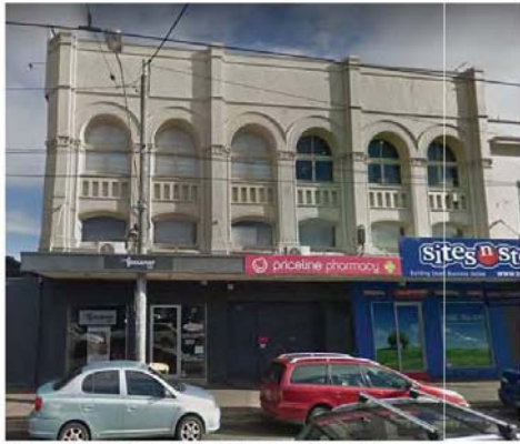
Figure 7. 252 Church St, Richmond (Google)
