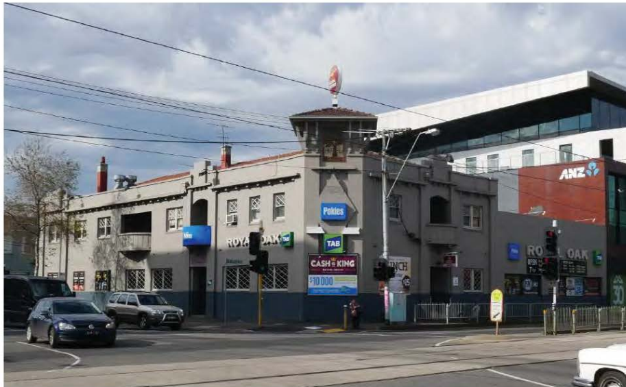
Figure 1. 529-533 Bridge Road, Richmond (GJM Heritage, September 2017)
