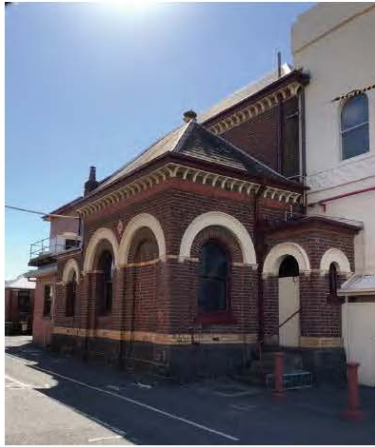
Figure 12. Junction of 1869-71 building and 1934-36 remodelled front façade, as evident on the west elevation.
