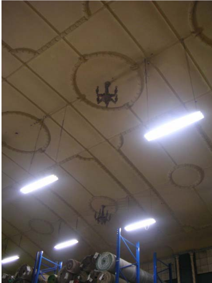
Part of the plaster ceiling in the main auditorium, 2004
