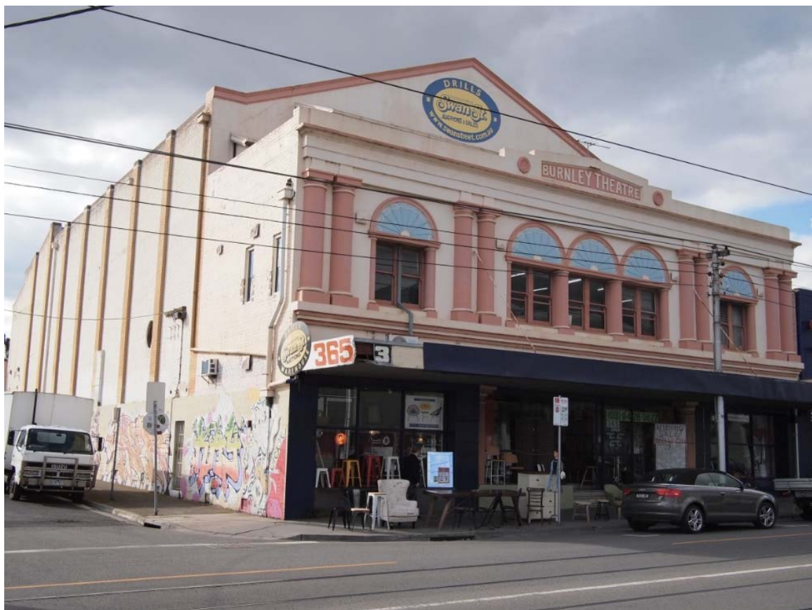
Former Burnley Theatre, 365 Swan Street, Burnley (Source: Context Pty Ltd, 2015)
