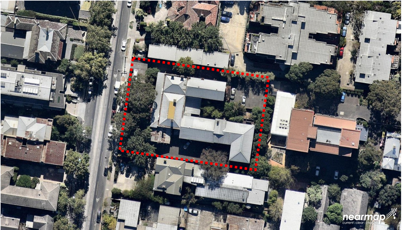
Figure 1: Aerial photograph - 351 Church Street, Richmond outlined in red (@nearmap, 4 April 2018)
