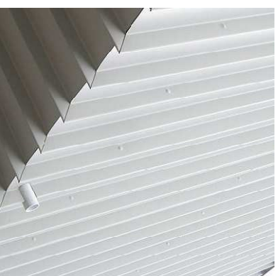
STANDING SEAM METAL CLADDING
