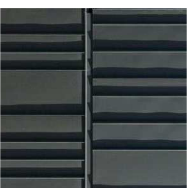
STANDING SEAM METAL CLADDING
