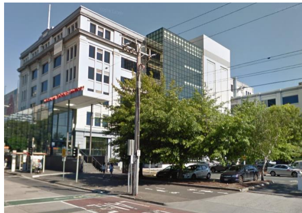
Picture 4 – Victoria Pde building – east elevation return
