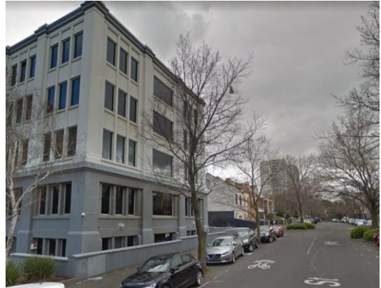
Picture 6 – Napier Street façade – more regular
