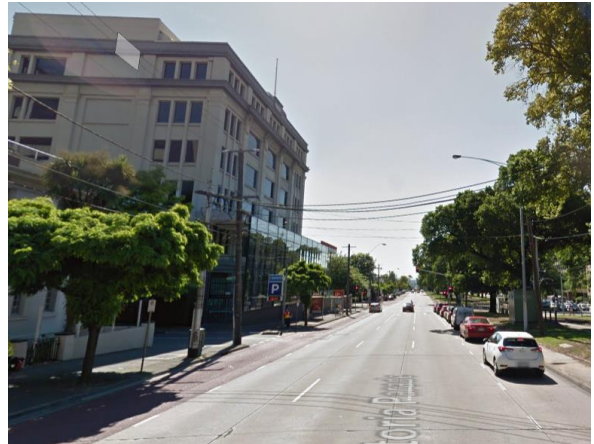
Picture 2 – West façade (close) from Victoria Pde
