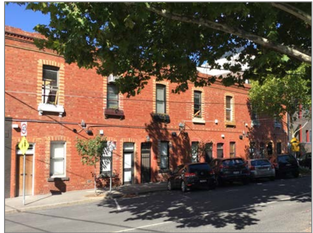
Figure 13. Cambridge Terrace, 50-62 Cambridge Street (HO336)
