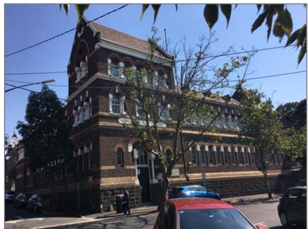
Figure 11. former Cambridge Street State School, 19 Street Cambridge Street (HO336)
