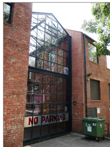
Figure 11. 1984 glazed link on Turner Street
