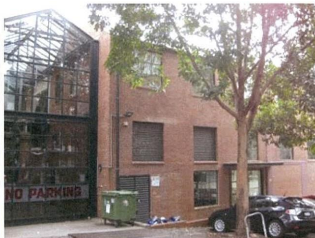
Figure 3. The 1920s factory building (right) and 1984 two-storey glazed structure that links the 1920s and 1911 buildings.
