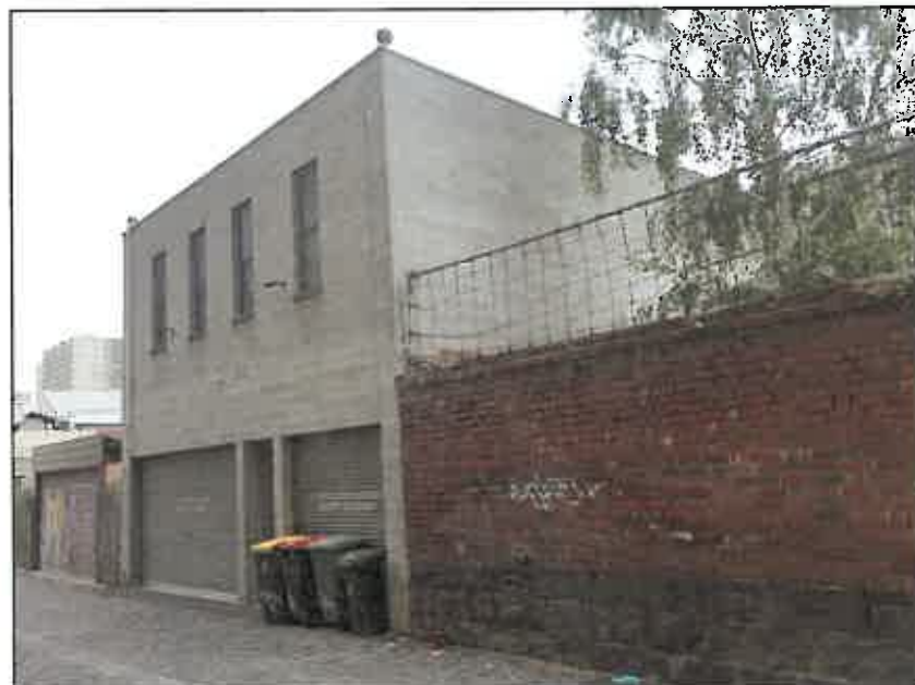
Figure 13 View of the western boundary from the south west, showing the high bluestone and brick wall to the rear of the adjacent property at 9 Brunswick Street.
