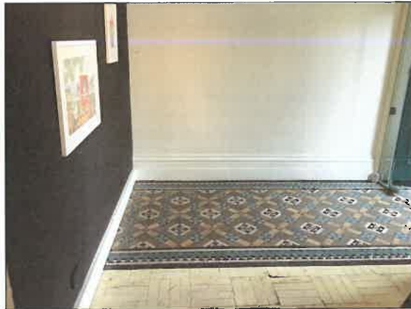
Figure 16 View to the front entry portion of the tiled entry hall, and the partition that separates this area from the stair beyond. This partition is to be removed.
