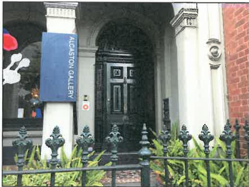
Figure 6 The Brunswick Street facade retains its original configuration of openings, including the original front door joinery.
