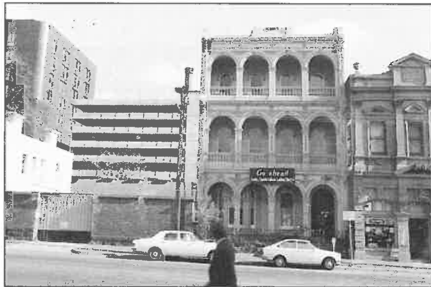
Figure 3 A c.1970s view of 11 Brunswick Street, showing the original parapet to have been truncated by this time.
