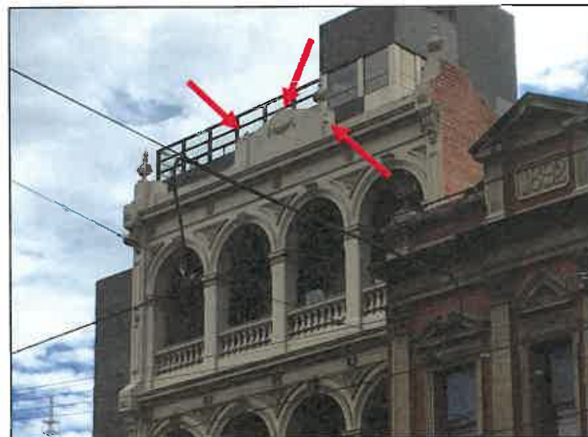
Figure 9 Arrows indicate the remaining evidence of the original balustraded parapet, the location where a parapet urn is missing, and the pediment in its present abbreviated form.
