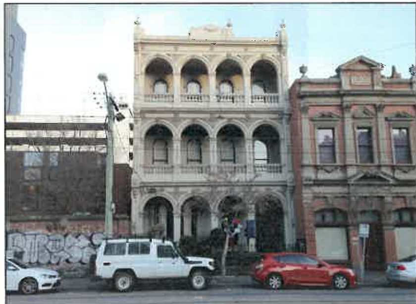
Figure 5 Existing view of the Brunswick Street frontage of 11 Brunswick Street.
