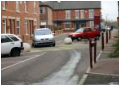
Northmoor Home Zone, Manchester
