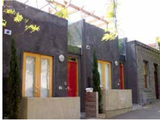
Courtney Street, North Melbourne
