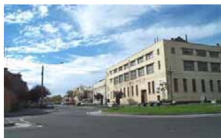
Warehouse buildings in West Melbourne Example of a Precinct undergoing change.
