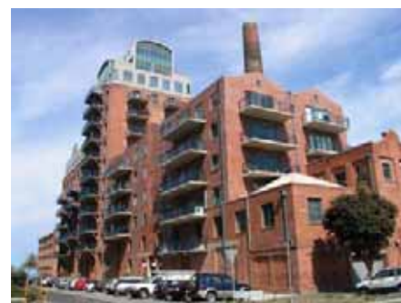
Sandridge Bay Tower - Old Starch Factory, Beach Street Port Melbourne
