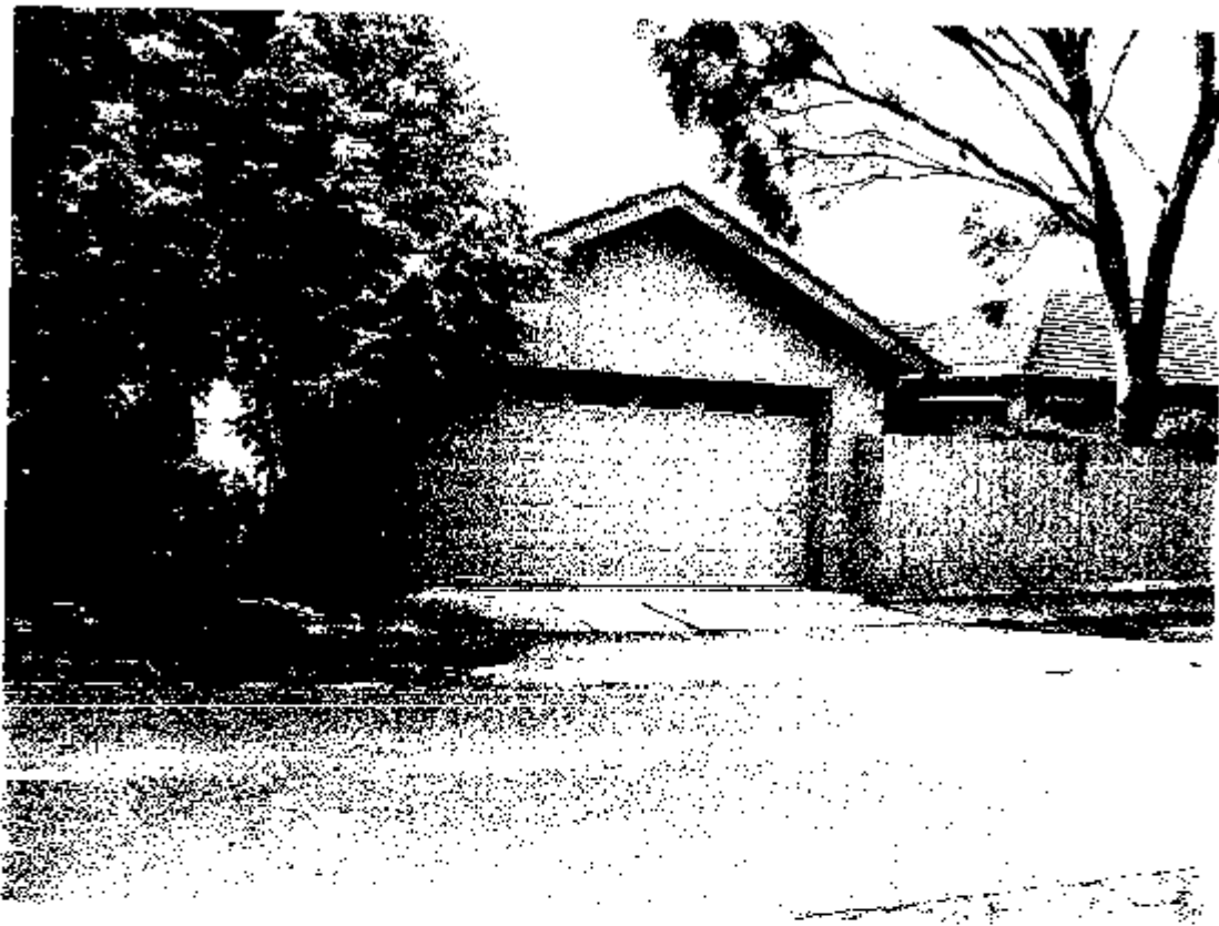
View of 9 Park Avenue showing the recent garage located over the Road. The northern (left hand) wall of the garage approximates the northern boundary of the Road.
