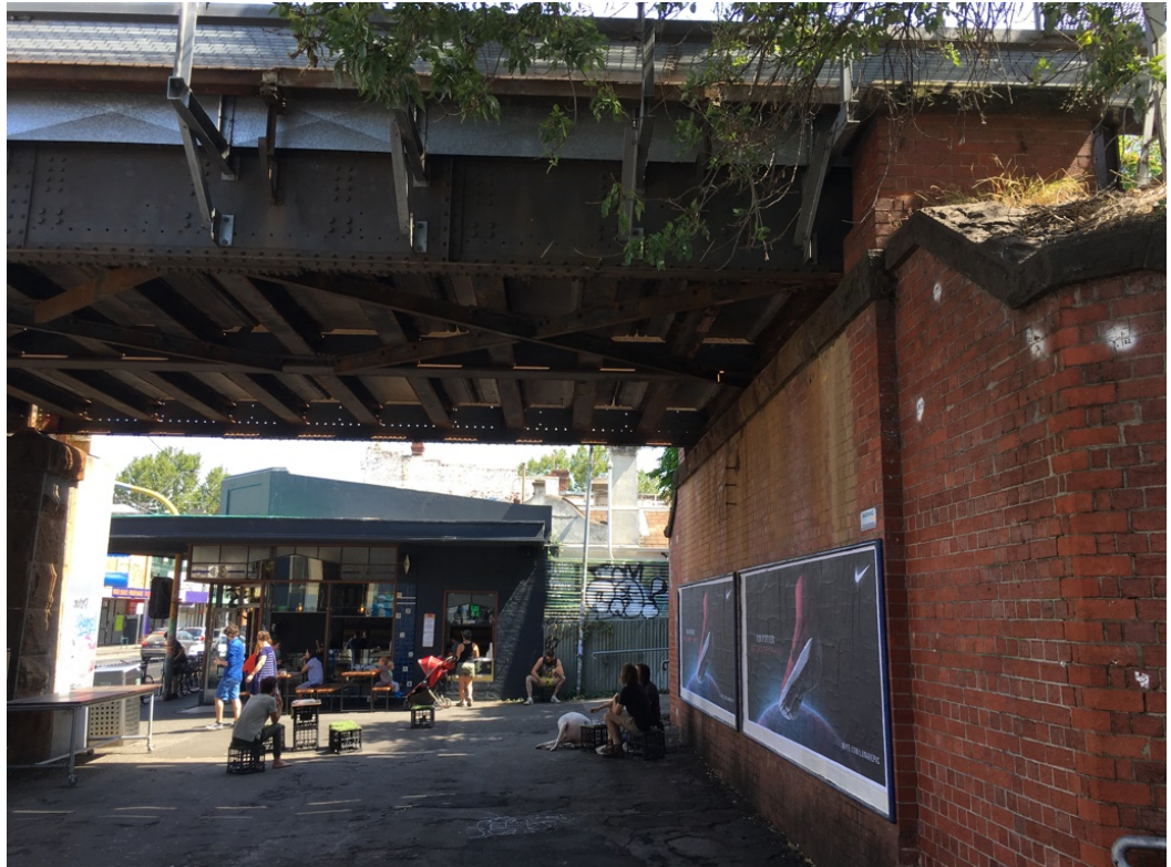
Railway bridge abutments, north side, looking through to no.274 Johnston Street
