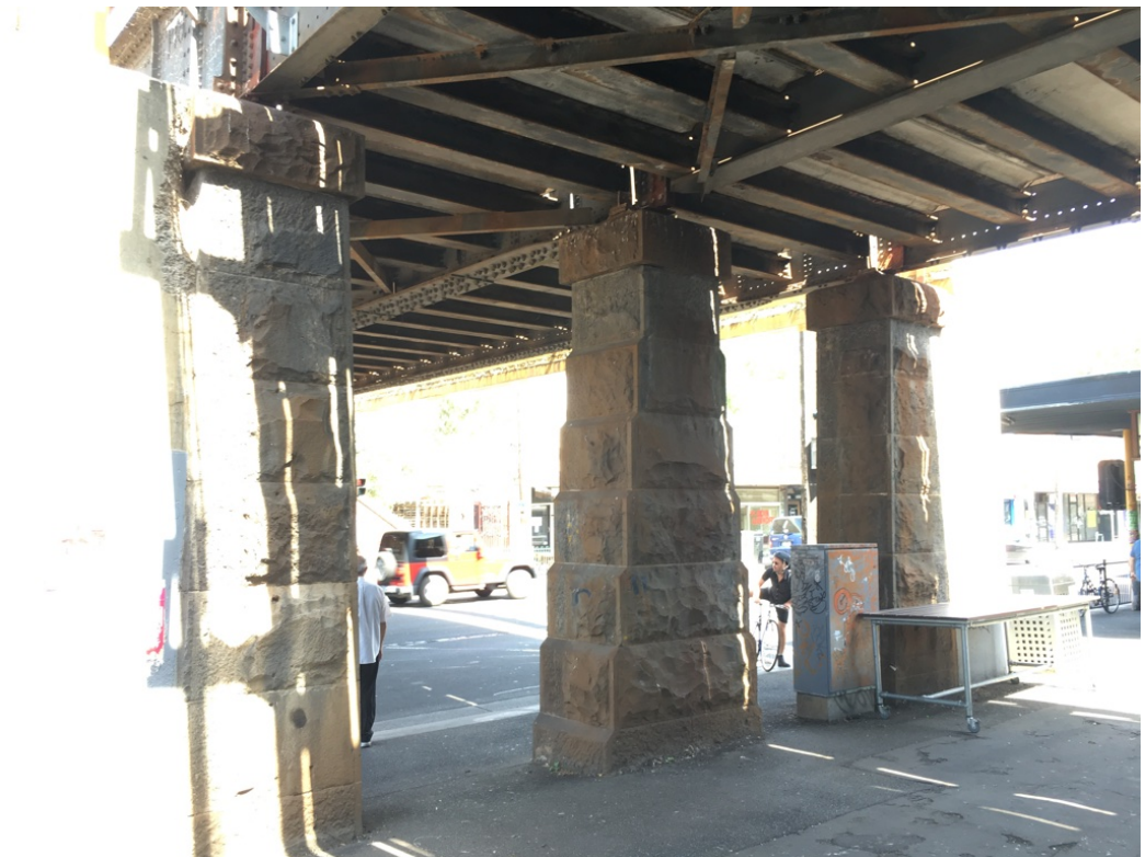
Tapered stone piers on the north side of Johnston Street
