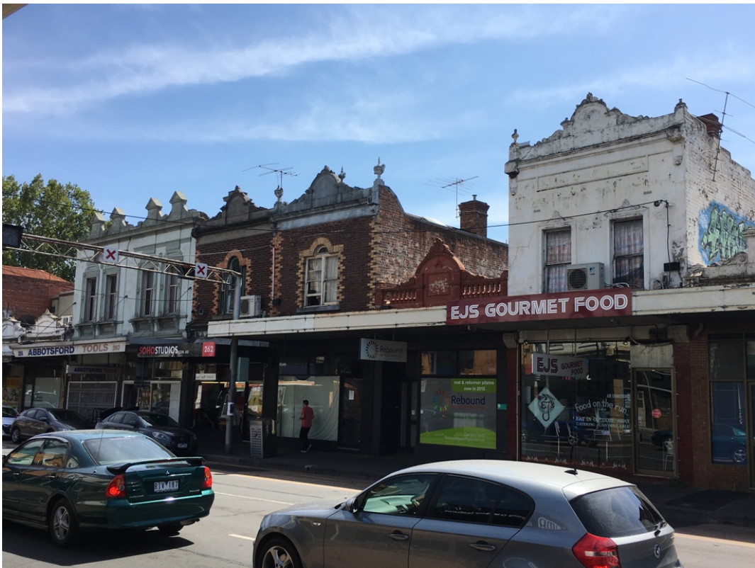
Johnston Street, north side looking west showing (from left to right) nos. 258-50, 260-62, 264 & 266
