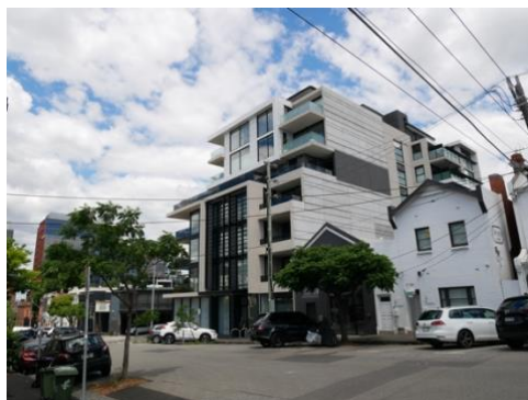
Figure 18. (left) North side of Derby Street looking towards the subject site (indicated) from the intersection with Oxford Street (nos. 10-22 Derby Street subject to HO102)
