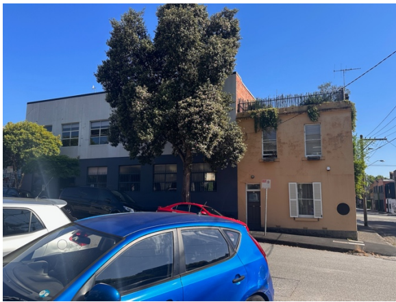
Figure 04: Subject site, Derby Street frontage, with adjoining heritage house at 8 Derby Street, and Little Oxford Street at right.
