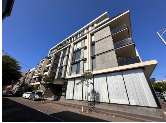
Figure 19: Development at 19-21 Derby Street (corner Oxford Street).
