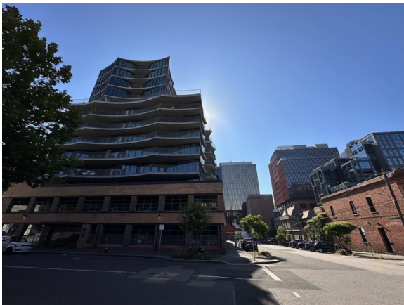
Figure 16: Development at 61-71 Wellington Street, viewed looking east across Cambridge Street towards Wellington Street, with Derby Street at right.
