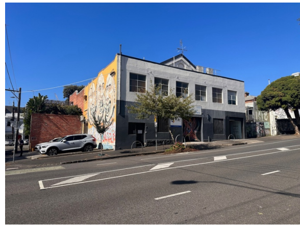
Figure 05: Subject site, Langridge Street frontage, with Little Oxford Street at left.
