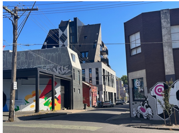
Figure 08: Contemporary development on Little Oxford street, looking north from Langridge Street.
