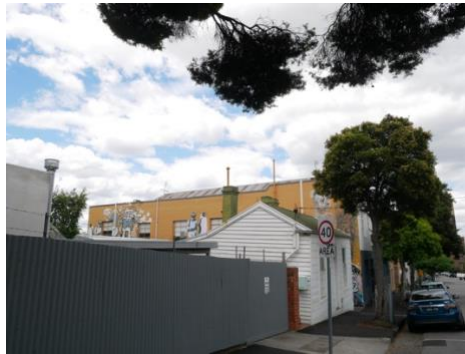
Figure 11. (left) Looking north along unnamed laneway from Derby Street along western boundary of subject site.
