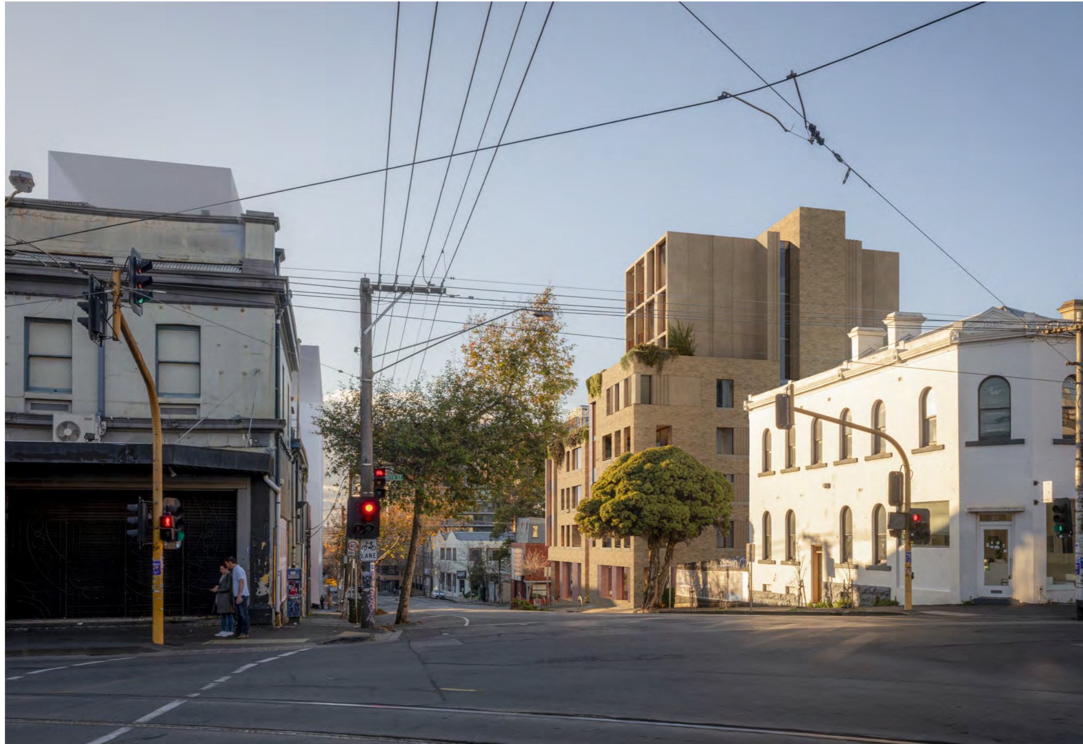
View from the corner of Langridge Street and Smith Street - Including Proposed Developments
