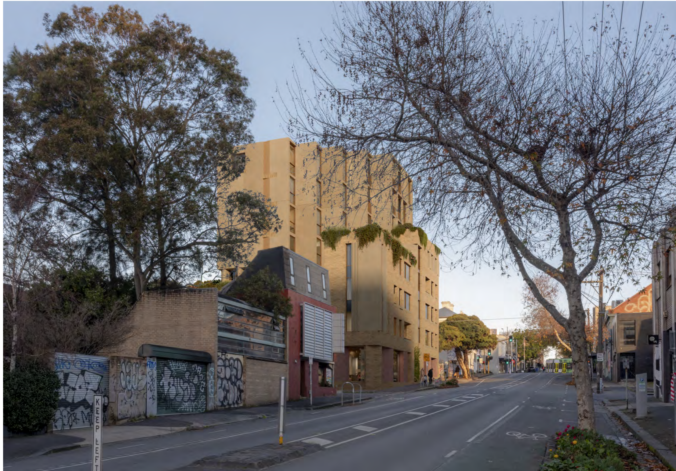
Local Context Design Response : Langridge Street View Towards Smith Street- Excluding Proposed Developments
