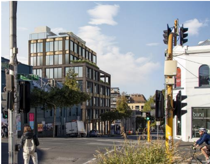
Image 14: perspective render of the approval at 4 – 12 Langridge Street as viewed from across Smith Street (WPP as circulated at VCAT for PLN20/0470)
