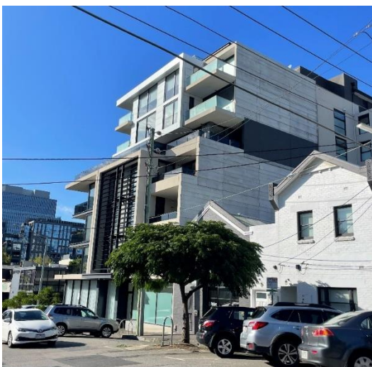
Image 10: the development as it appears from the west along Derby Street (Officer site visit, April 2024)
