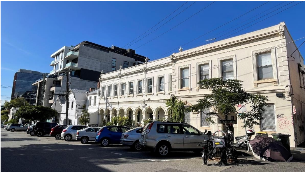
Image 19: development on the opposite (south) side of Derby Street (Officer site visit, April 2024)
