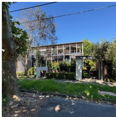
Figure 5: Adjoining property at No. 11 Arthur Street
