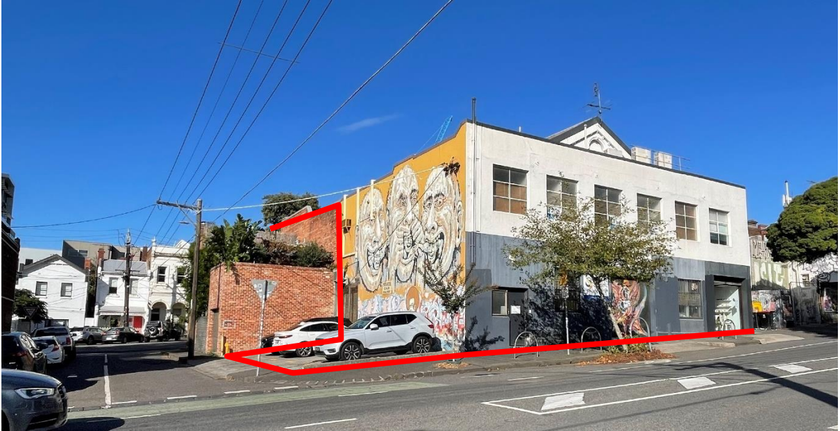
Image 8: the subject site as seen from the north-east from Langridge Street (Officer site visit, April 2024)
