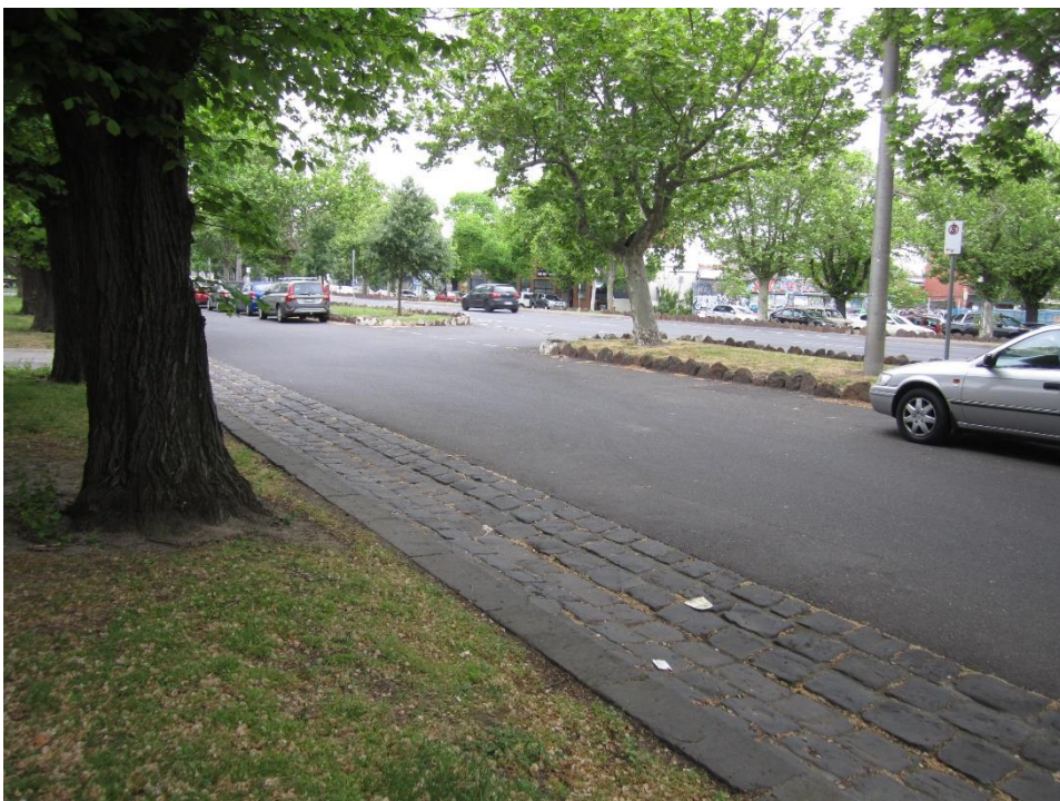
Figure 13: Type 3 curb and drainage channel.
