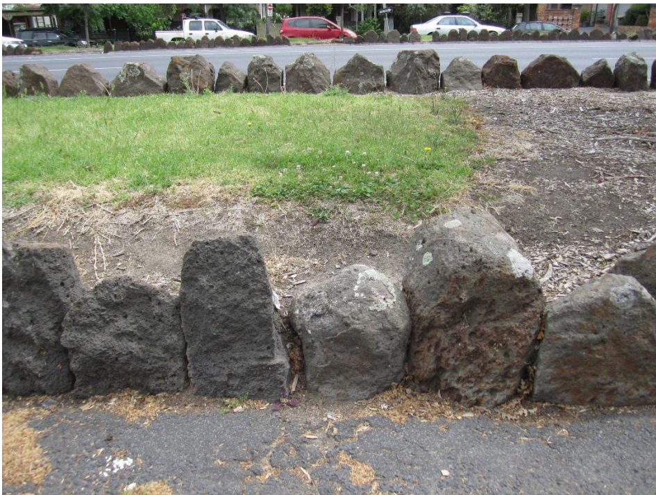
Figure 8: Uncut basalt blocks form a prominent and decorative border to the medians. This remnant fabric is remarkably intact.
