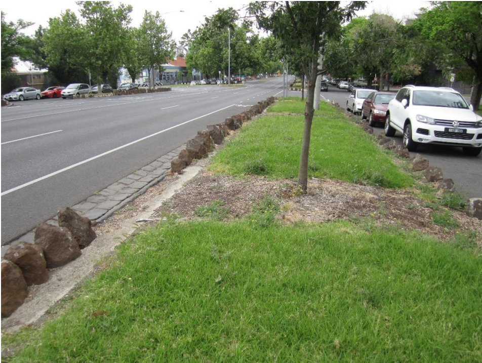
Figure 9: Median immediately north of Jamieson Street. A portion of the row of uncut basalt blocks toward the central traffic lanes is absent in two locations, apparently associated with tree planting. The concrete base toward the central lanes is visible at left of frame.
