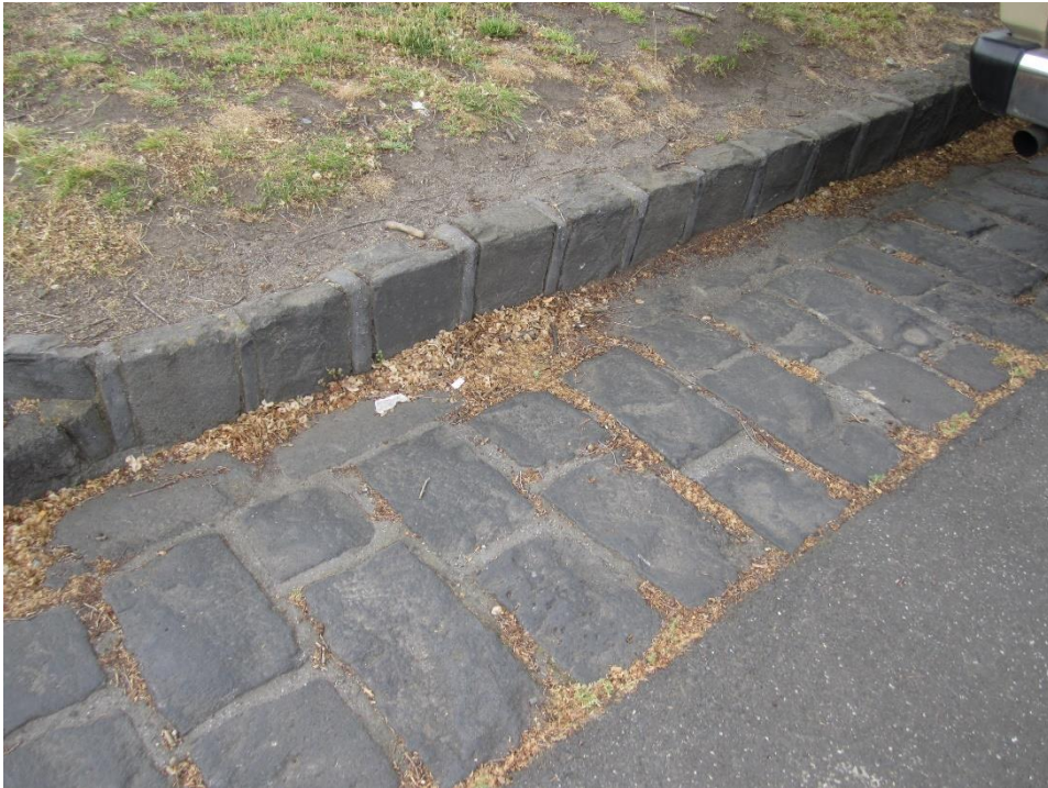
Figure 17: Type 7 curb and drainage channel.
