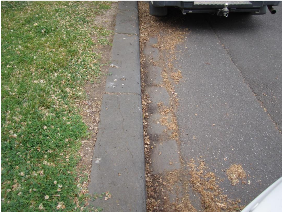
Figure 12: Type 2 curb and drainage channel.
