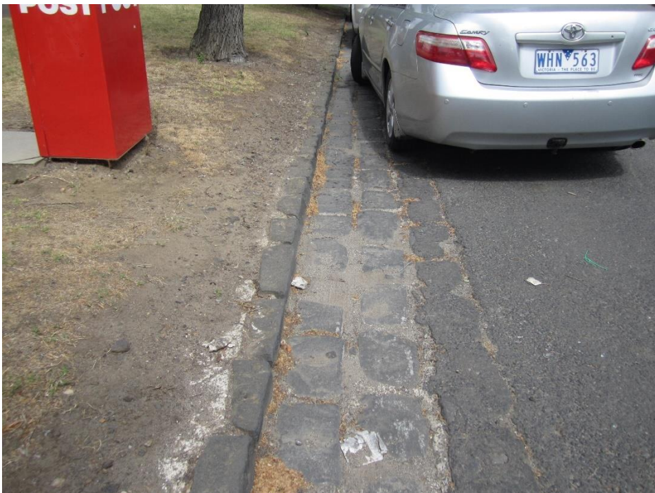
Figure 16: Type 6 curb and drainage channel.
