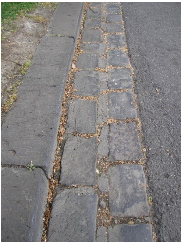
Figure 14: Type 4 curb and drainage channel.
