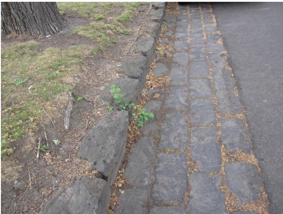
Figure 18: Type 8 curb and drainage channel.
