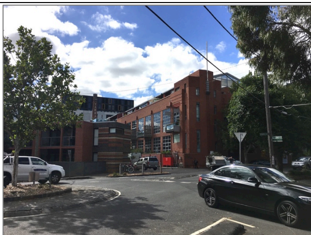
Byfas Ltd Factory – 8-16 Trenerry Crescent, Abbotsford (HO314 – Yarra Falls Precinct) *Note: land surrounding the art deco building is not within the HO
